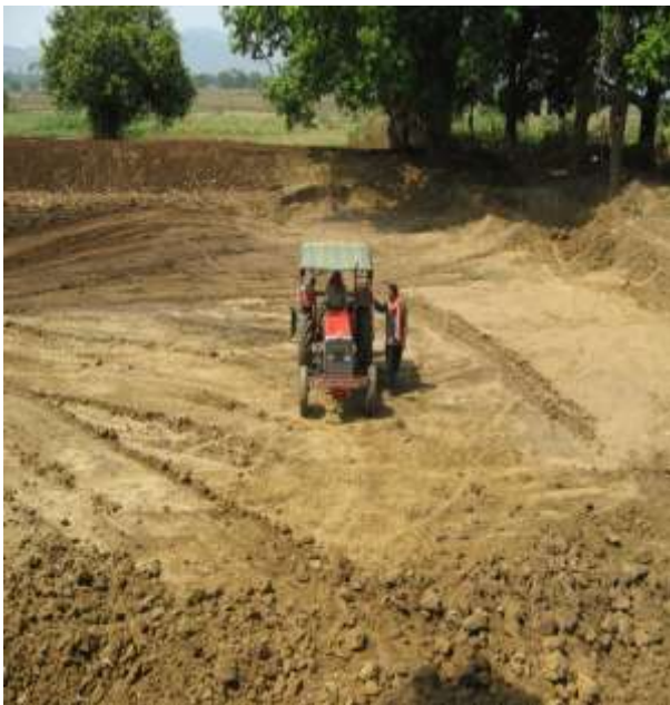
Construction of pond for prawn culture
